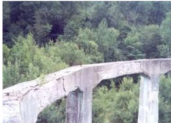
Rappel Shot: Anonymous source saw rungs for securing a propulsion device for the Bell.
